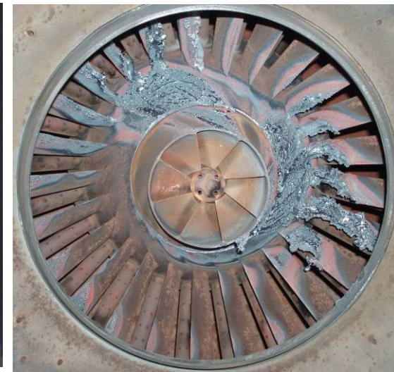
Damage Caused by Flash Back
